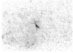
Coating damage can appear as gouges, cracks, and punctures. Hail-induced coating cracks often form patterns shaped like "crow's feet" or semicircles.
