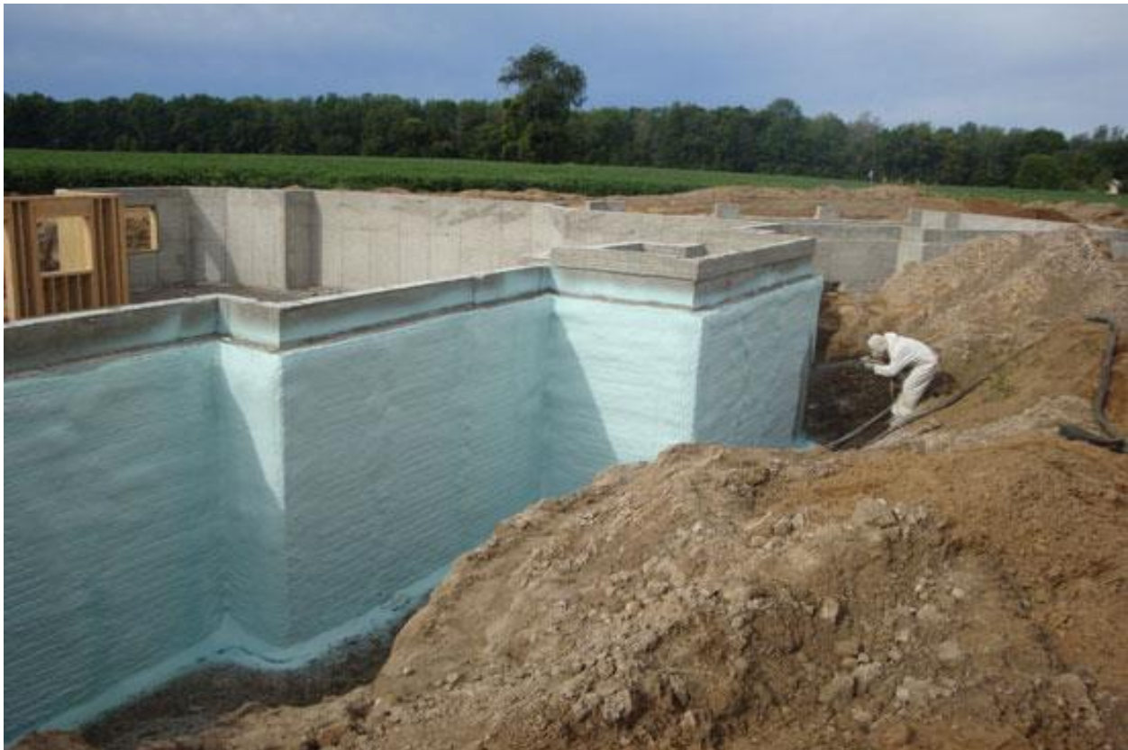
Figure 3 – Exterior below-grade wall installation (photo)
