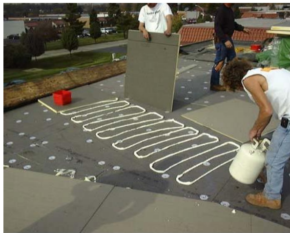
FIGURE 4: SPF ADHESIVE RIBBON APPLICATION
