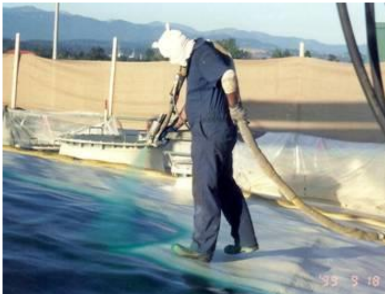
Figure 11: Spraying a fast curing, plural-component coating onto SPF
