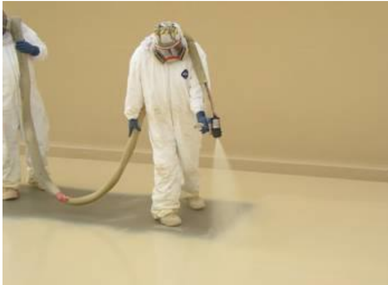
Figure 10: Spraying a fast curing, plural-component coating onto concrete
