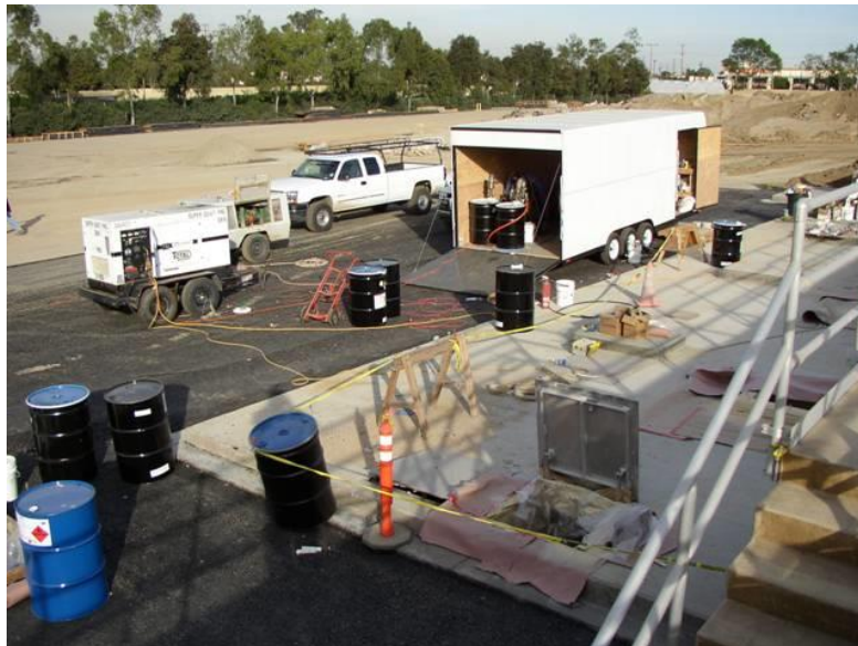
Figure 9: Typical field staging and setup
