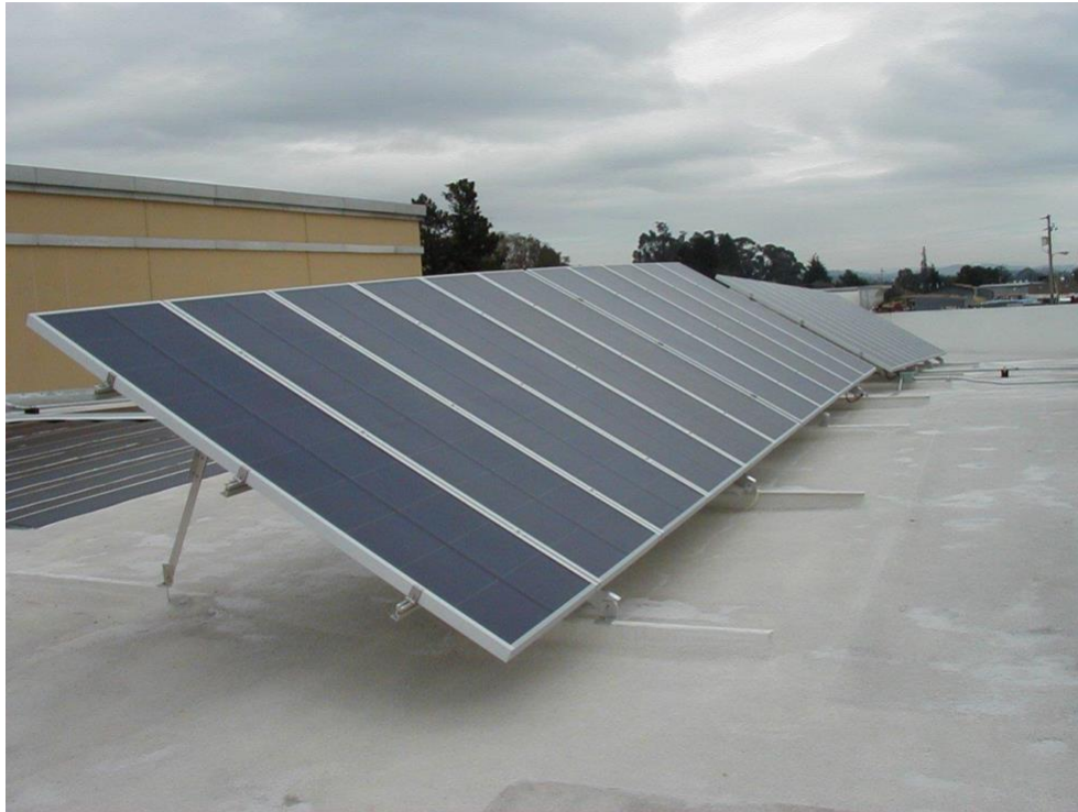
Figure 8 - Typical roof curb with truss supports.
