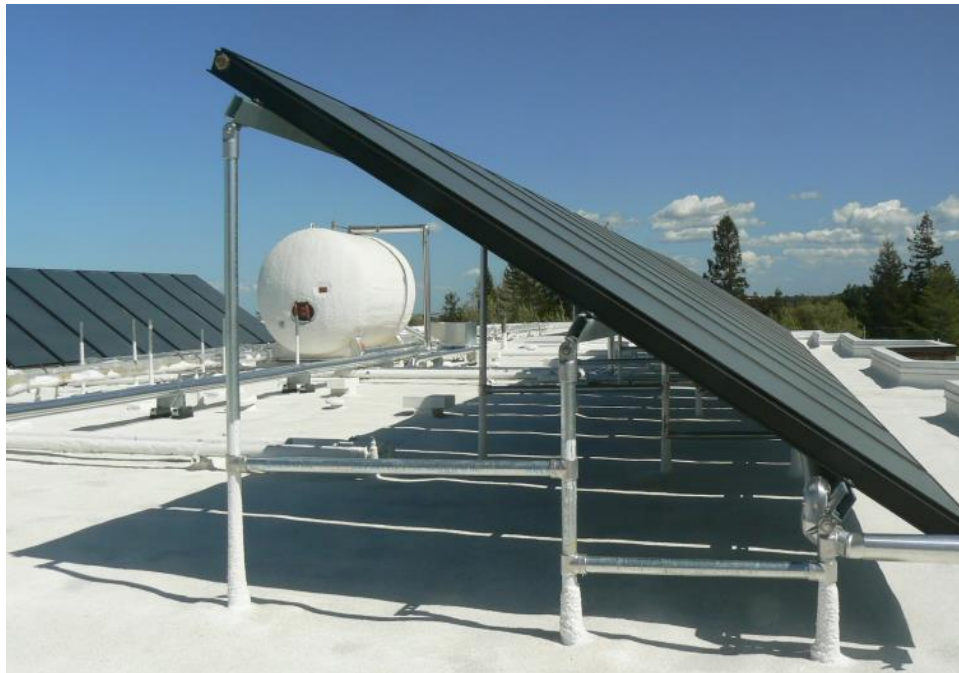
Figure 13 - Flashed stand-off attachment.
