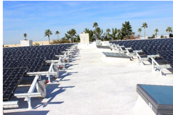
Figure 10 - Penetrating attachments with post/beam.
