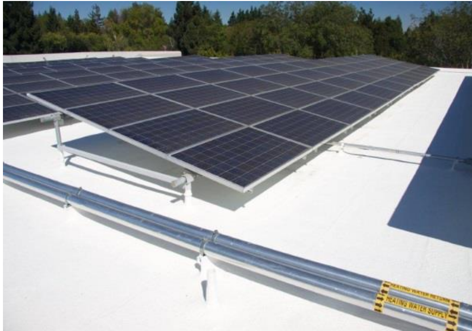
Figure 1 - Typical Penetrating Rack-Mounted PV System
