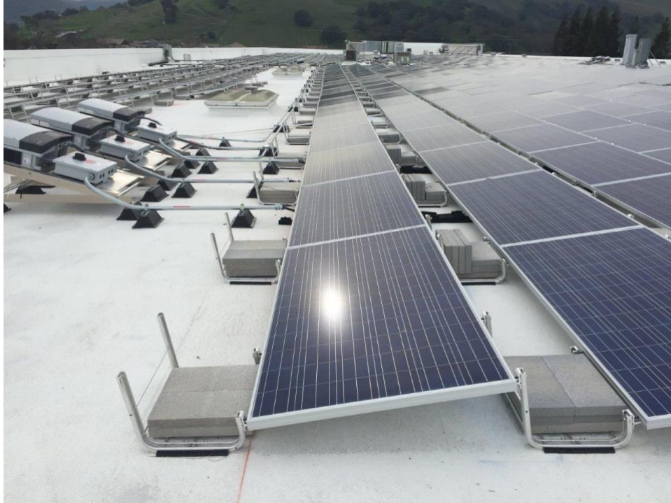
Figure 12 - Non-penetrating, ballasted system
