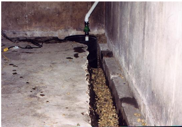
Figure 1 – Interior Foundation Drainage System with Sump Pump
