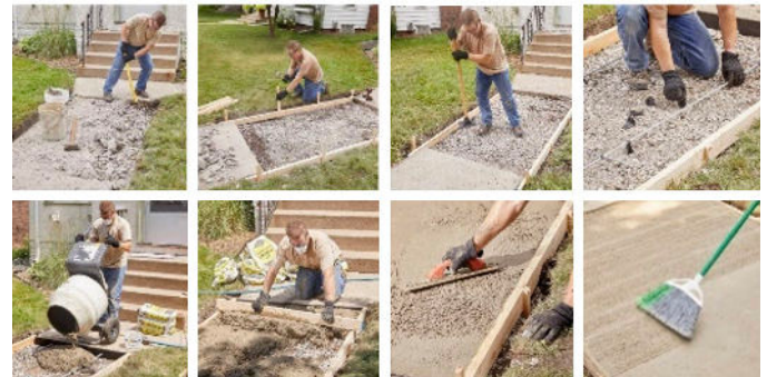
Concrete removal and replacement
